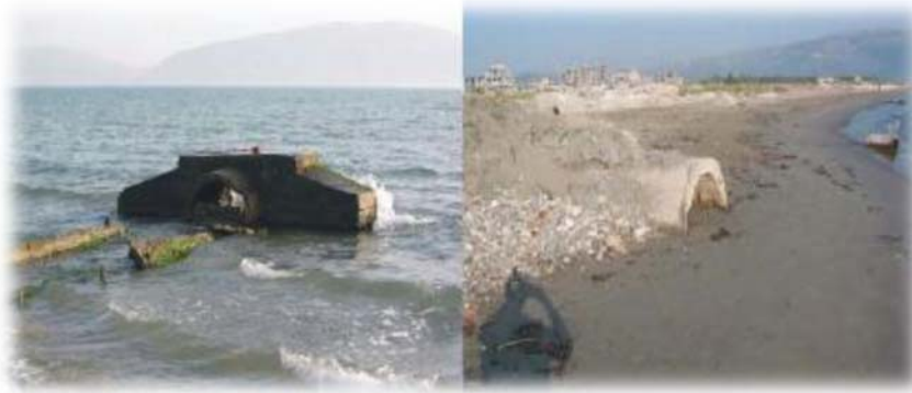
Figure 2 Direct discharges of waste from the Soda-PVC plant near the Gulf of Vlora.
